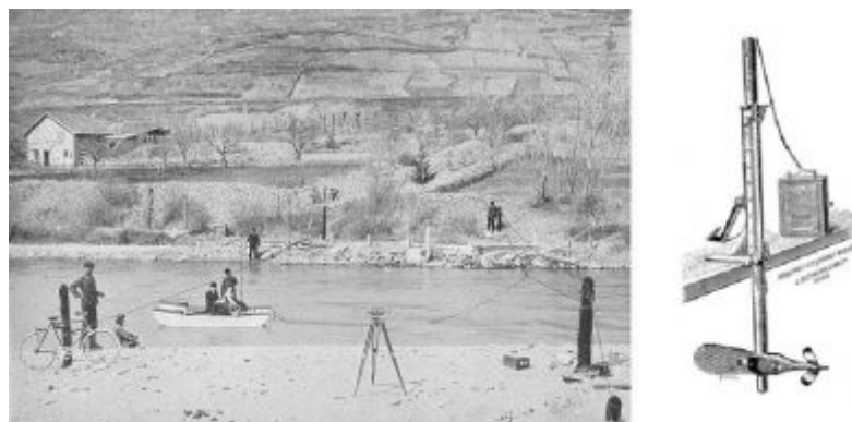
Figure 5. Gauging by exploring the speed field on the Durance at Embrun (Hautes Alpes) in 1910; on the right, Woltman principle reel of the "Richard" brand used from the boat.
