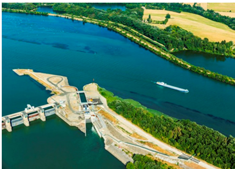
Figure 8. Small Hydropower Plant and fish passes at Rochemaure - Commissioning 10/2015 [Source: © Camille Moirenc]
