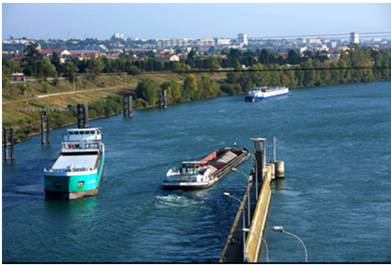
Figure 5. Lock entrance [Source: © Camille Moirenc]
