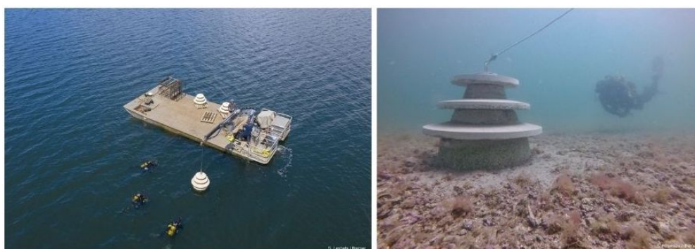
Figure 13. Restoring the former oyster beds of the past: implantation of concrete shell reefs in order to favour recruitment and revitalise the flat oyster populations of the Roz bank in Brest bay and the Penthievre bank in Quiberon bay. [Source: © IFREMER / Stéphane Lesbats (left) & Stéphane Pouvreau (right)]
