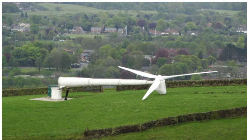
Figure 3. Wind turbine generator fall at Mount Etna, near Norden, Rochdale, UK [Source: © Colin Park, CC BY-SA 2.0, www.geograph.org.uk/ ]
