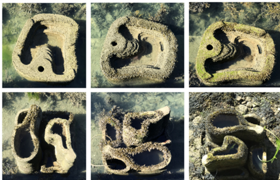
Figure 8. Case study of ecological rehabilitation in the port-Haliguen (Quiberon): installation of different tidal pool prototypes with significant 3D complexity. [Source © Seaboost - M. Lapinski]
