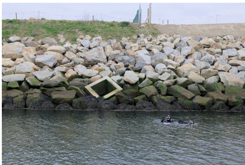
Figure 4. Example of an eco-block installed in the dike of the port of Brest (Bretagne-France). These eco-blocks remain filled with water at low tide, artificially recreating puddles characteristic of the rocky coasts of tidal seas. [Source © Ifremer - O. Dugornay]
