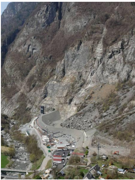
Figure 8. Protection barriers. [Source: Gavet, photo Sage]
