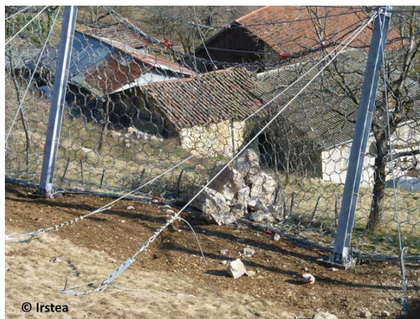
Figure 9. Deformable nets, Ripailler. [Source: IRSTEA]
